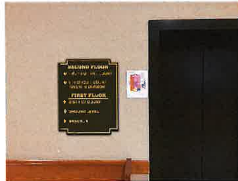
1/8" THICK ACRYLIC PANEL w/ RAISED GOLD LETTERING & BORDER MOUNTED FLUSH TO WALL
