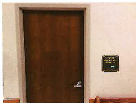
1/8" THICK ACRYLIC PANEL w/ RAISED GOLD LETTERING & BORDER, RAISED BRAILLE & (2) WITH SLIDER FOR ROOM USAGE, MOUNTED FLUSH TO WALLS
