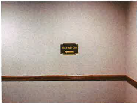
1/8" THICK ACRYLIC PANEL w/ RAISED GOLD LETTERING & BORDER, RAISED BRAILLE, MOUNTED FLUSH TO WALL
