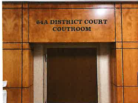
3/8" THICK ACRYLIC LETTERS w/ SATIN PAINTED FINISH MOUNTED FLUSH TO WOOD
