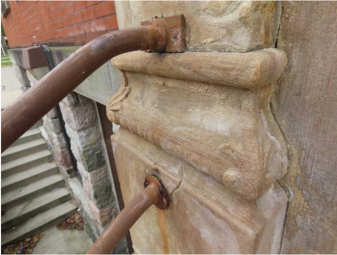
North Elevation Steel Handrail Attachment at Stone
