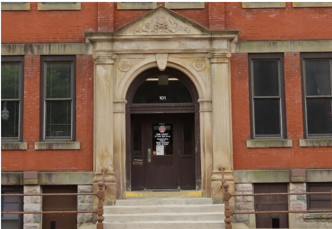
North Elevation Front Entry – The front entrance is surrounded with ornate, Classically detailed sandstone.
