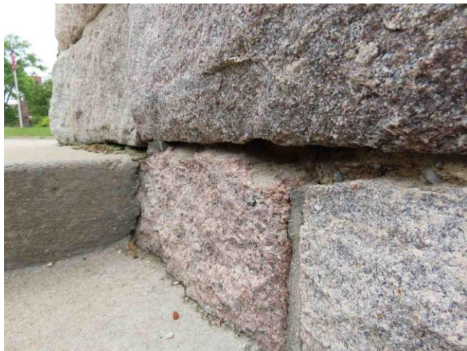
North Elevation Mortar Joint, Typical
