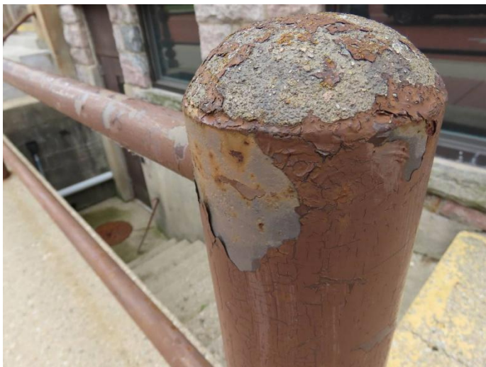
North Elevation Steel Railing Post, Typical
