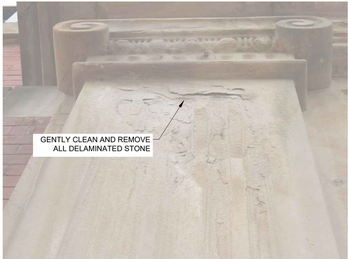
1.4 Sandstone Detail, Typ.
