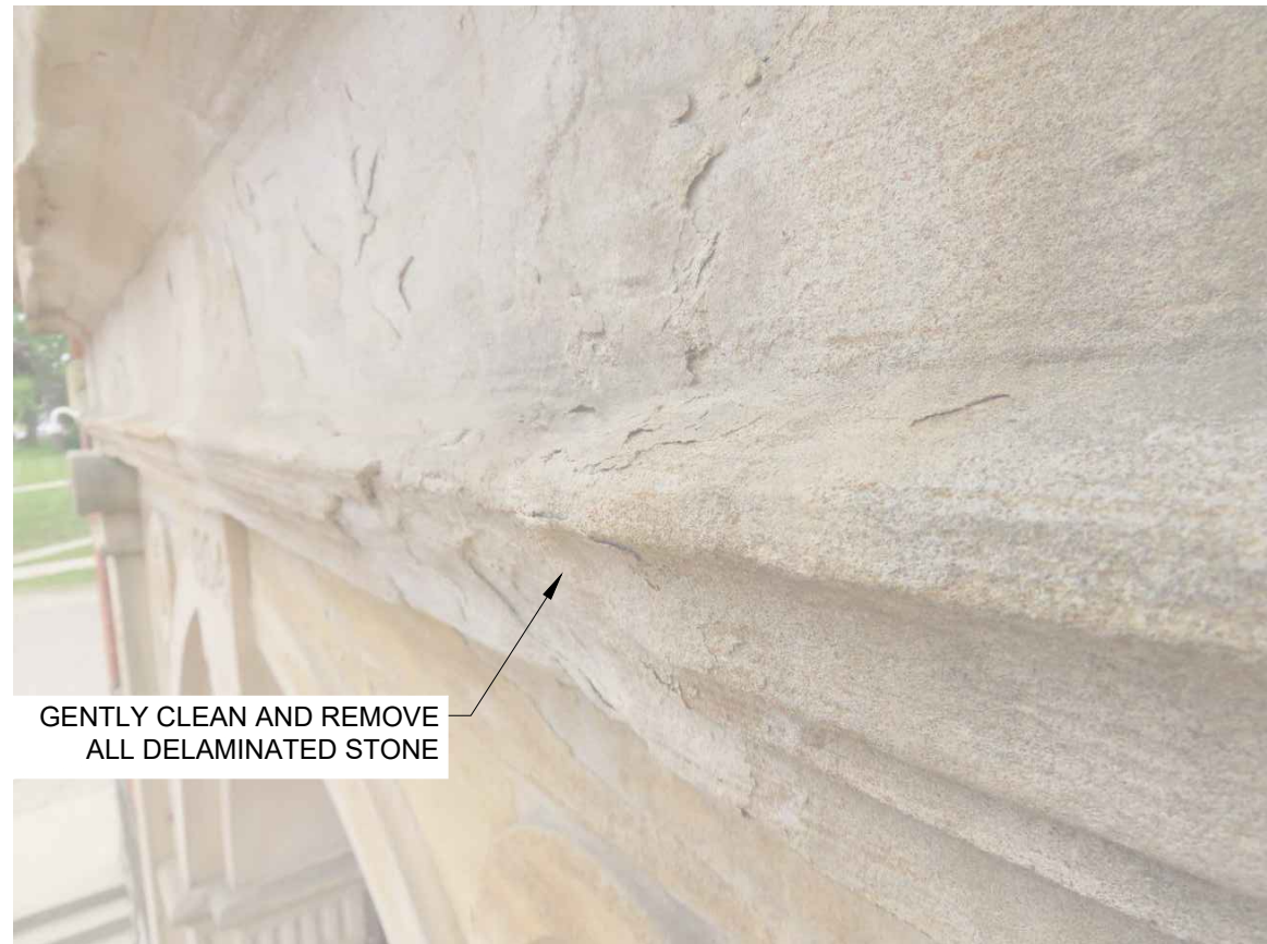
1.3 Sandstone Detail, Typ.
