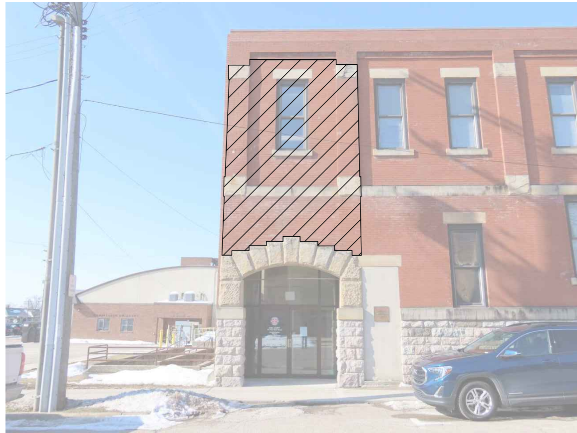
1.1 Item 2 - Area of Work
