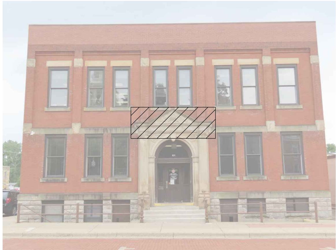
1.1 North Entrance Pediment - Area of Work
